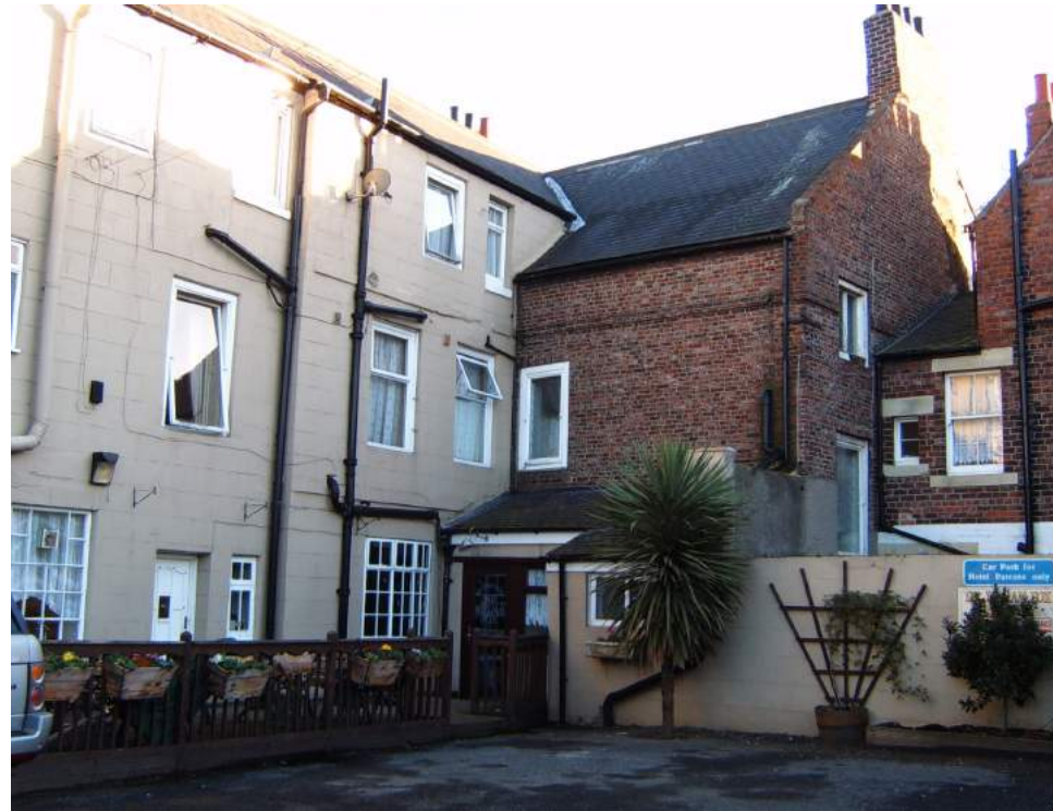
JUNCTION BETWEEN EARLY AND LATE GEORGIAN BUILDINGS
