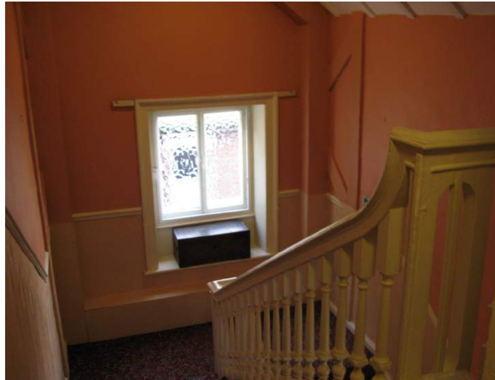
VIEW OF THE EXISTING STAIRCASE
